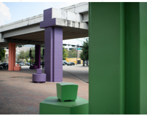
↑ Milam / Spur 527 Underpass
